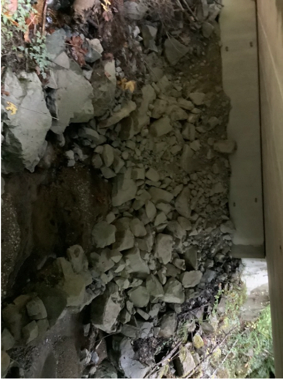
Left Bank Abutment when facing downstream
