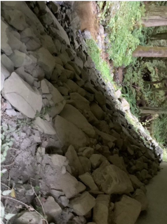
Right Bank Abutment when facing downstream
